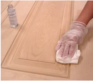
Step 1: Clean door with mineral spirits, rinse.
