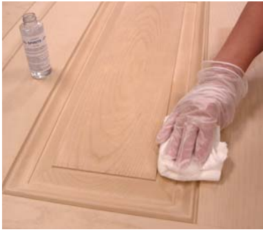
Step 1: Clean door with mineral spirits, rinse.
